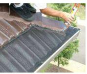
Step 8: Then seal with silicone into place. To prevent the mesh from lifting.
