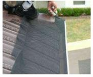
Step 5: To avoid damage to pointing or bedding, we stop tucking the mesh about three tiles from the end of the run. The mesh is then cut around the profile of the
