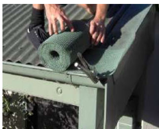
Step 1 : Mesh is clamped to beginning edge of gutter.
