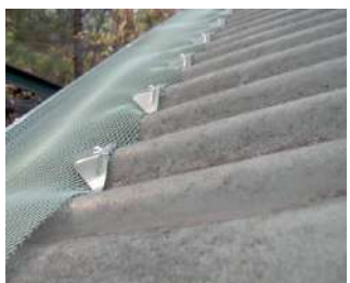
Step 4 : Saddles are screwed on every second corrugation.
