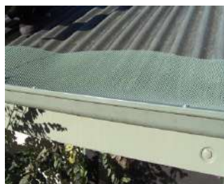
Step 2 : Trim is fixed to gutter lip
