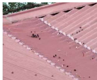
Step 6: With a valley a 250mm or 500mm wide mesh can be used. It is simple rolled out and fastened on every corrugation on either side of the valley with saddles.
