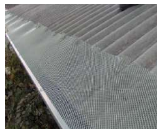
Step 3 : Mesh is then slit every second corrugation. The slit is along each side of the corrugation and should not exceed 20mm.
